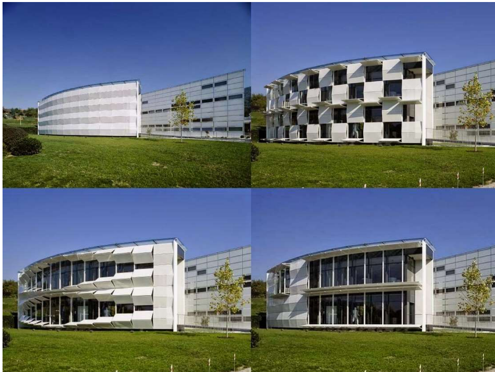
Fig. 1: Kiefer Technic Showroom
